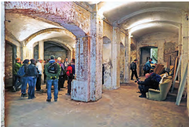
The extensive ice cellar (or Pestkeller) we visited. The two methods of vaulting can be made out
